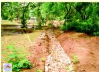
Stream intervention with in situ stones leading to rain gardens after 10 h of rainfall of 57 mm in 3 h at NGRI
