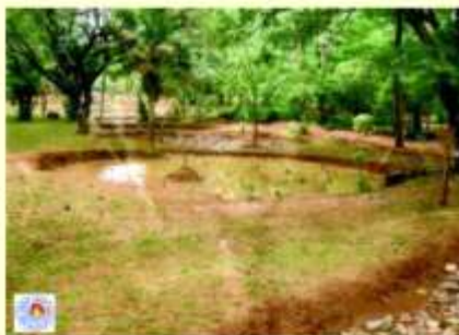
Rain gardens with Water ponding after 57 mm of rainfall for 3 h (9-12pm) on 14 July after 10 h of the rainfall at NGRI
